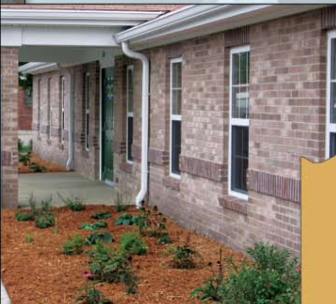
Newton Village in Kentland, Indiana, was awarded a $70,000 grant in the second round of 2005 through Lafayette Bank and Trust Company, NA, in partnership with CDC Resources, Inc. This new construction project using the HUD-811 Program and AHP created six rental units that serve very low-income individuals that have developmental or physical disabilities.
