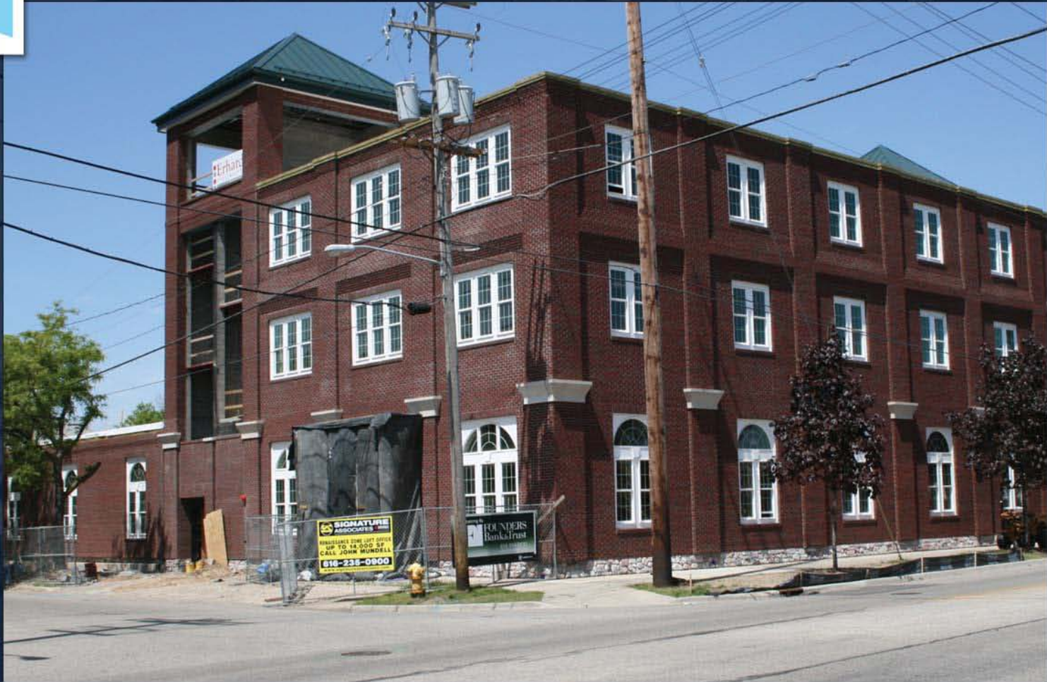
Drueke Building, Grand Rapids, MI CIP advance: $3.4M - job creation, neighborhood revitalization Member: Founders Bank & Trust
