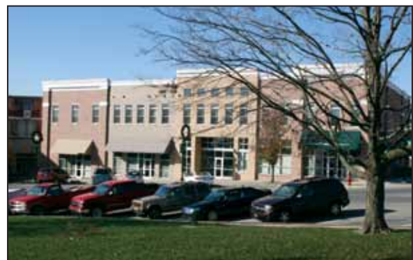
Out of the ashes of a devastating fire rose the Phoenix on the Square in downtown Paoli, IN. Retail space occupies the first floor facing the courthouse square with affordable apartments in the back and on the second floor. Hoosier Uplands Economic Development Corp. was awarded an AHP grant of $750,000 through Old National Bank.
