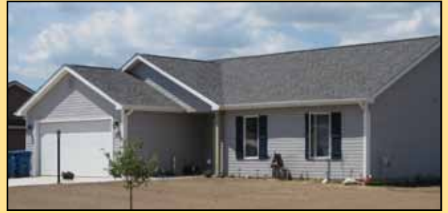
Dogwood Estates in Walkerton, IN was financed with a variety of funding sources, including LIHTC, the federal Neighborhood Stabilization Program and a $556,750 grant from the FHLBI's Affordable Housing Program through FHLBI member 1st Source Bank.
