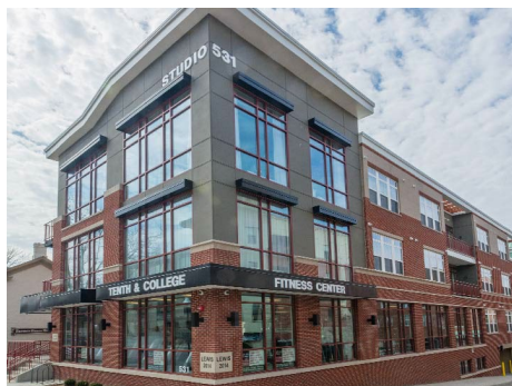
Market Rate Apartments in Bloomington renting for $1,900 for a one-bedroom unit
