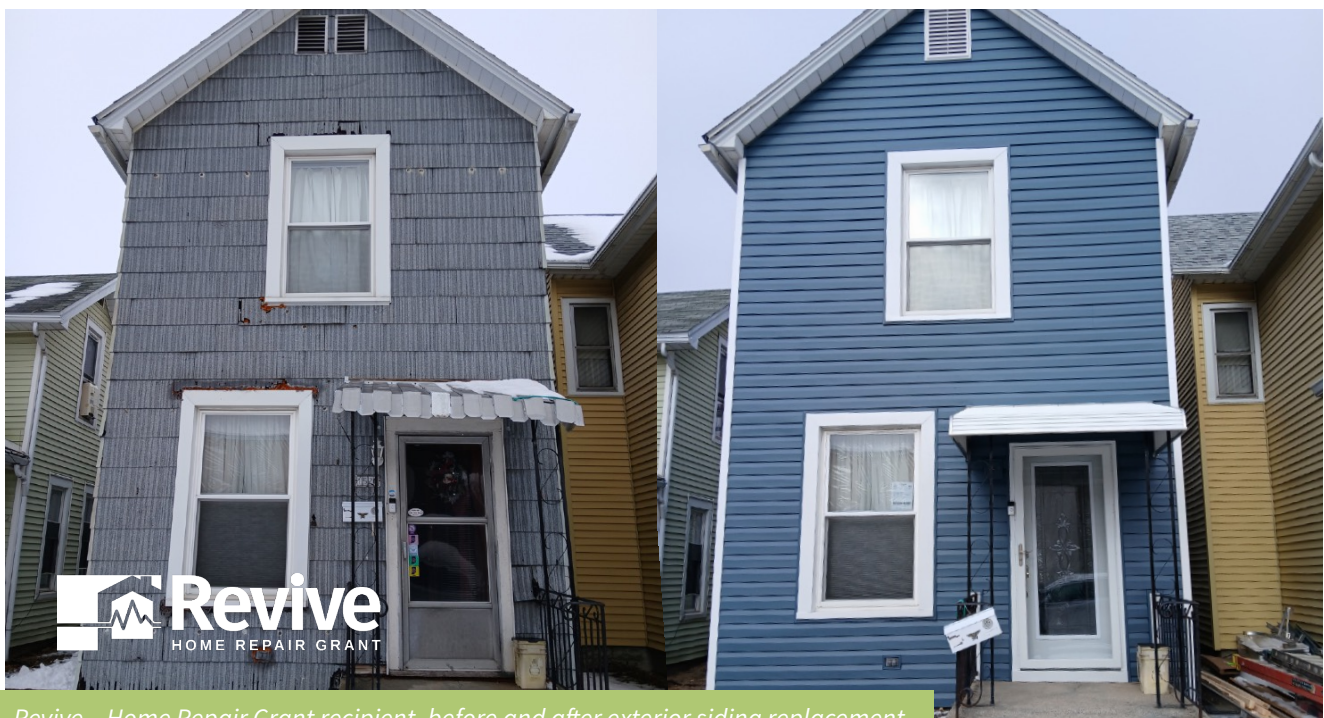
Revive – Home Repair Grant recipient, before and after exterior siding replacement
